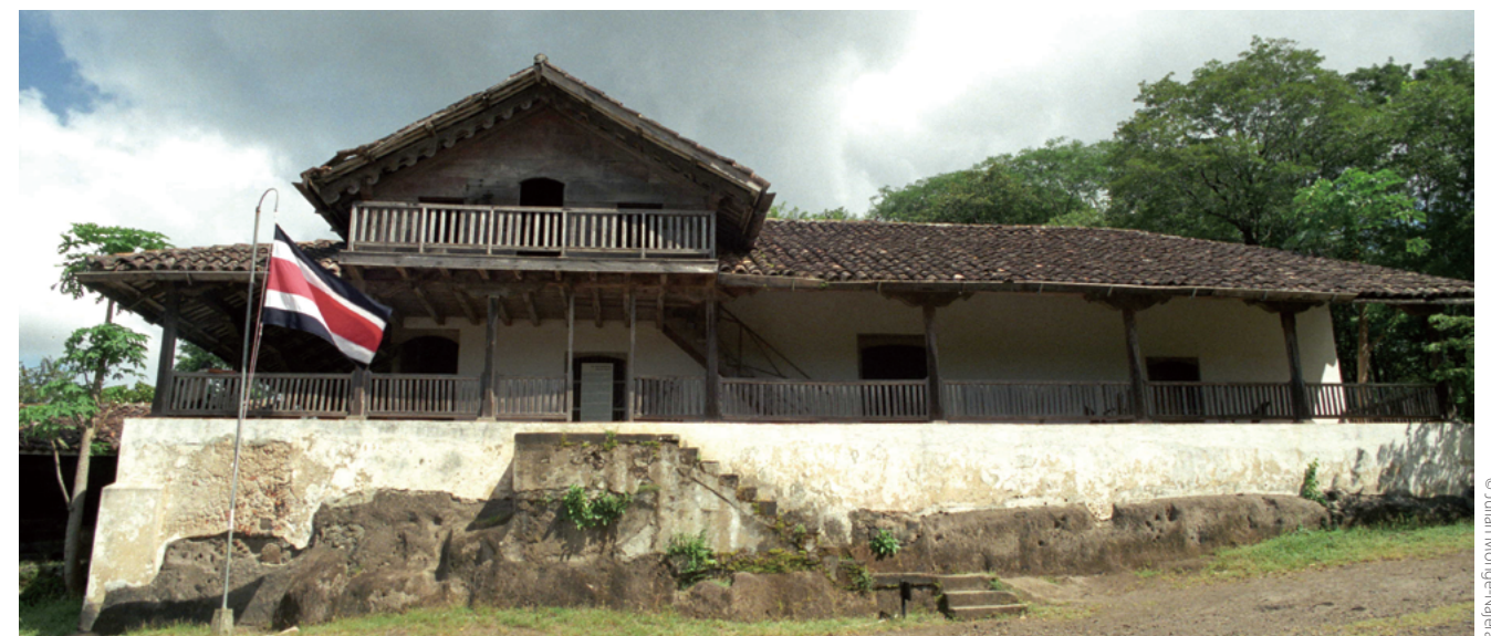
La Casona before the fire, 1999.
