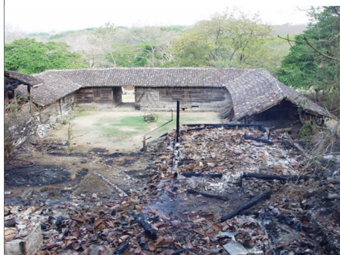
La Casona right after the fire.
