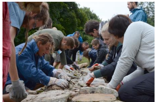
Figure 13 – Practical lesson in dry stone walling. International summer workshop / volunteer camp on Učka mountain, Kvarner-Croatia. Photo: Nevena Kereša
